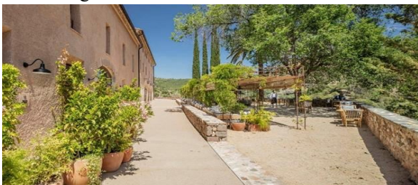
Figure 6. The scene after the reconstruction of the main entrance road of talk dominical hotel. (photo source: moue design network).
