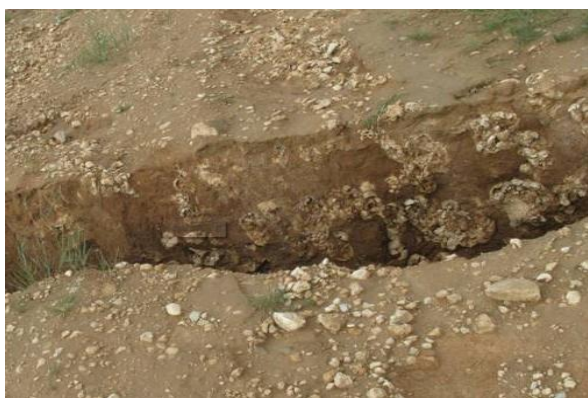
Figure 2. Ground cracks in the mining area.
