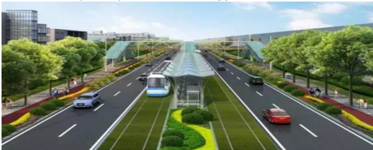
Figure 1. Achievements of a road construction in PPP project in X city.
